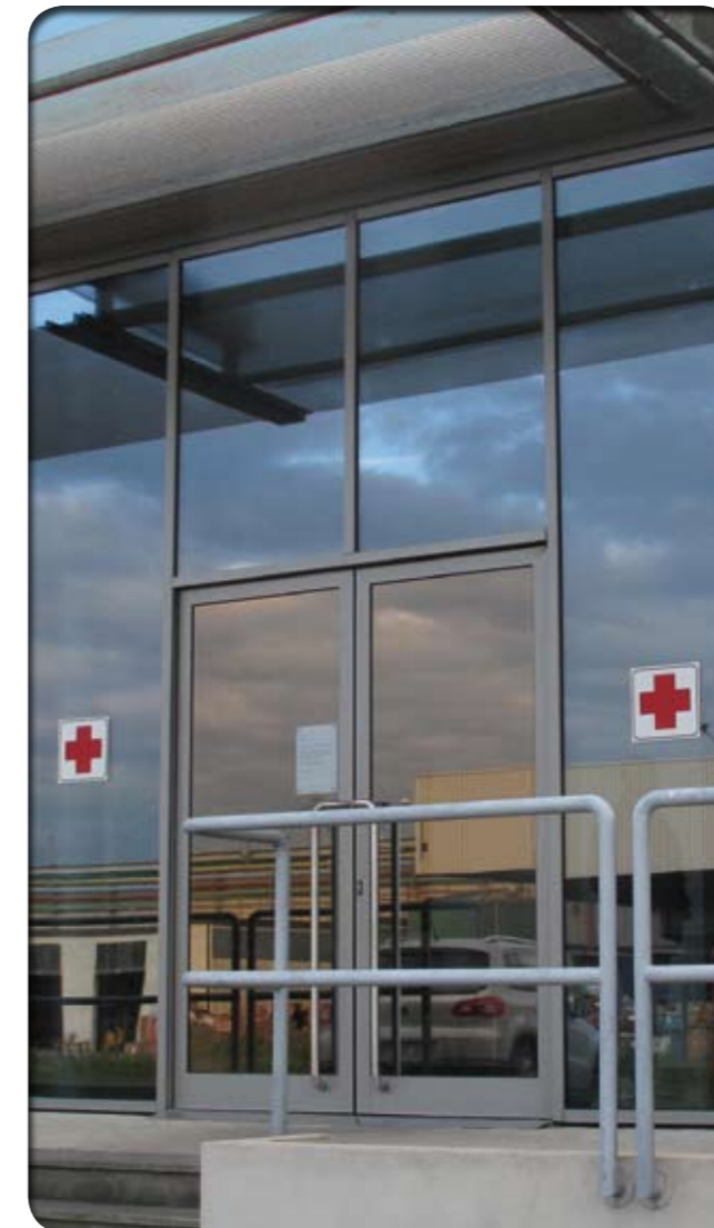
Company Medical Centre at Pontedera (Pisa)
